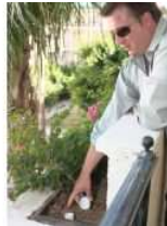
Jennifer Salman/Special to the AFN Ahwatukee Foothills resident Matt Schryver's company, Save Water Solutions, has installed a smart water harvesting system on the grounds at Arizona Grand Resort to help conserve water when watering plantlife.
